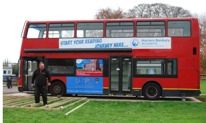
The Library Bus in position with new decking being installed.
